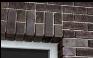
Window lintel perfectly replicated with angles.
