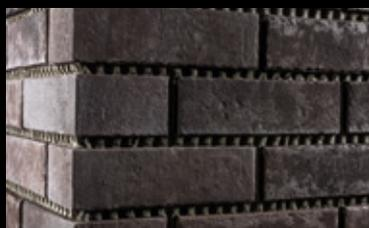
The finished surface. Grouting can be done after the appropriate drying time.
